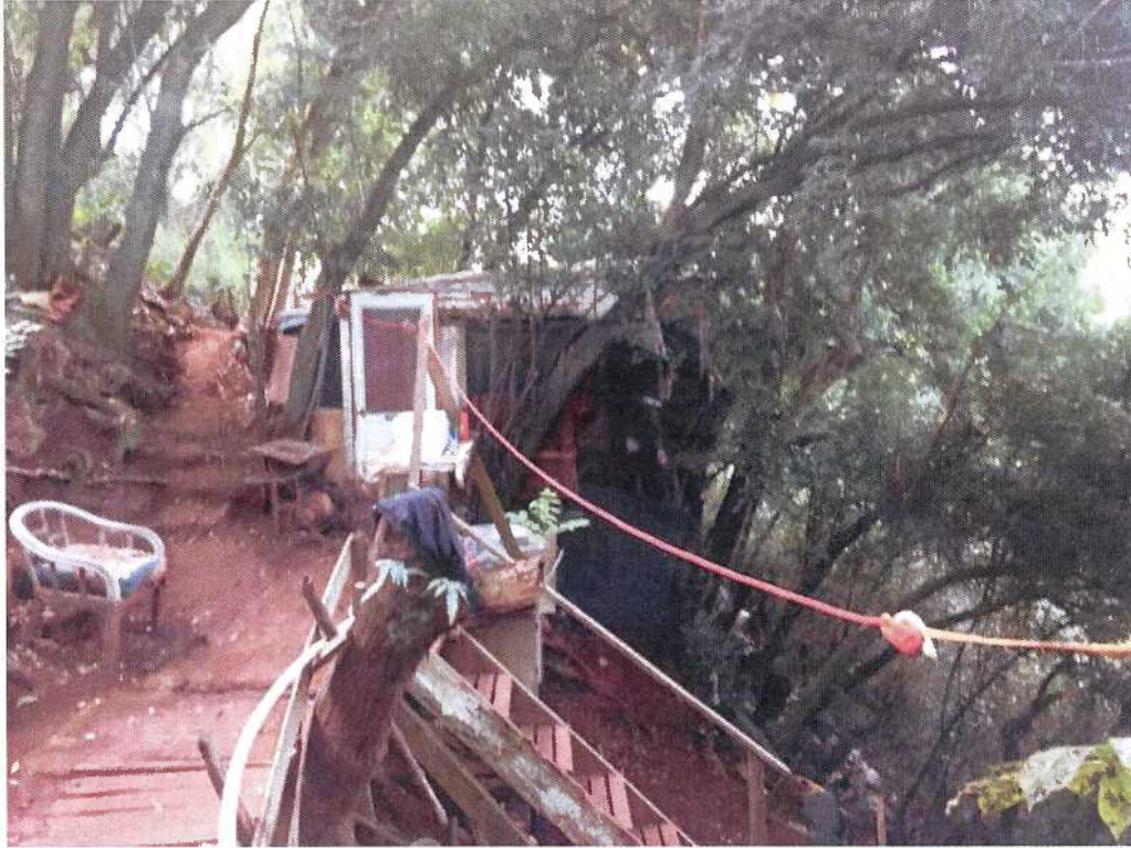
Illegal structure built on ADC property in natural forested area along Uwalu Circle
