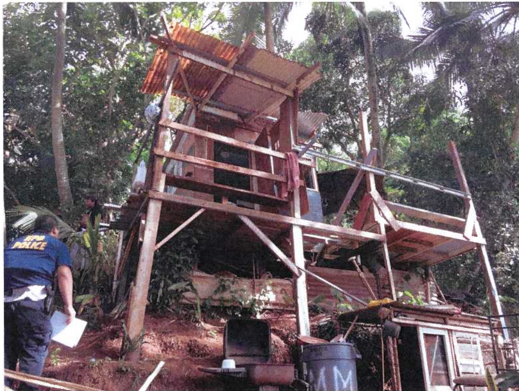
Illegal structure built on ADC property in natural forested area along Uwalu Circle
