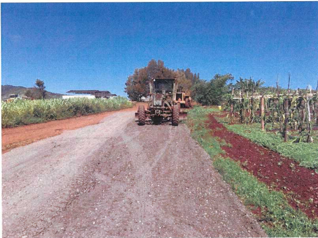
Crushed gravel being placed on the dirt road on September 20, 2018
