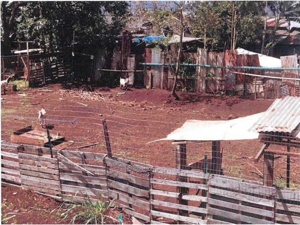
Goat pen within drainage easement on State property
