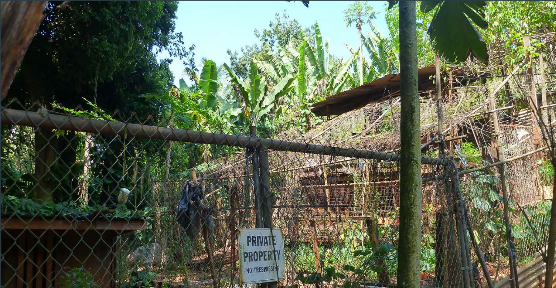
Fencing, structures, and chicken coops located on State property.
